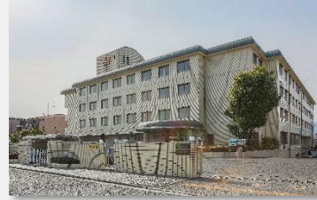
ElySION Mamigaoka & Annex
