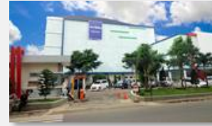
Siloam Hospitals Purwakarta
