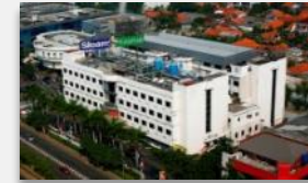
Siloam Hospitals Kebon Jeruk
